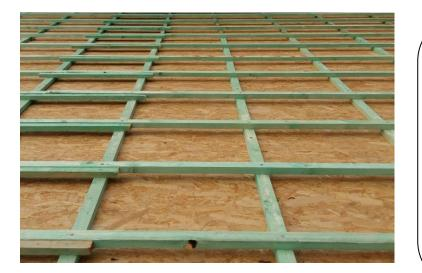
The **Cerasolpan** needs a tiling batten distance of **40.8** cm from top to top. After placing the tiling battens, tracing the distance of **35.2** cm between the Suntiles can be done. The counter battens need to be minimum 20 mm heigh for good ventilation and let the connectors go under the battens while connecting.
