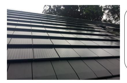
The electrical connection between the sun tiles is easy: just click in each other two MC4 connectors and connection is a fact! Each Sun tile has its own bypass diode, when failure of a suntile occurs, the string will not be interrupted.
