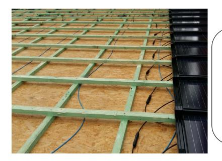
Now each column is traced at 35.2 cm we can prepare the solar cables (strings) on the under roof. One end will be connected to the string of the Suntiles and the other end of the cable to the Optimizers / inverter inside the building.
