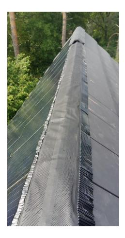
Through natural convection , the Suntiles are cooled. Therefore it's important to install a ventilated ridge.
