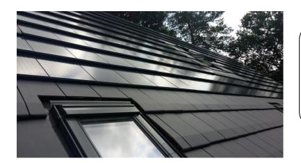
The further finishing of the roof can be in combination with the flat ceramic tiles from Terreal as the Volnay but also with the Tuile plat from Monier.
