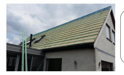
The Sun tiles from Smartroof are placed on a sloped roof such as the classic tile and can be installed during roof renovations and new constructions. No special underroof is needed.
