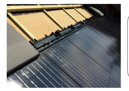
Each tile is fixed with a stainless steel screw on the tiling batten. An integrated hook makes that the tiles are holding nicely each other and making the roof homogeneous, airtight and weathers the storm. Total weight of the system is only 18 kg/m<sup>2</sup>!
