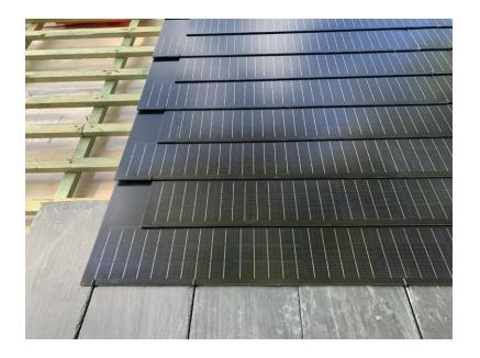
Each Sunslate is fixed with two stainless steel screws on the tiling batten. A specific hook makes that the Sunslates are holding nicely each other and making the roof homogeneous, airtight and weathers the storm. Total weight of the system is only 24 kg/m²!
