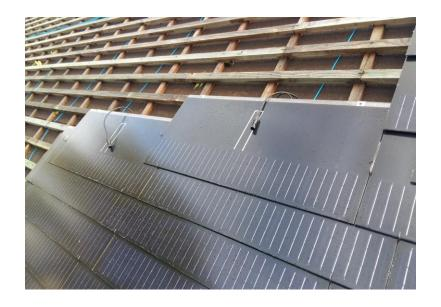
The electrical connection between the Sunslates is easy: just click in each other two MC4 connectors and electrical connection is a fact! Each Sunslate has its own bypass diode. If one Sunslate is defective, the string will not be interrupted!
