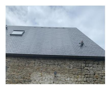
Finishing the roof can be in combination with the natural slates of Cupa, Samaca, Gaëlic, ... 40/22 but also with the synthetic slates New Stonit from Etex 40/24. Ventilation at the ridge is necessary to obtain a good natural convection of the underroof and cool down the Sunslates.
