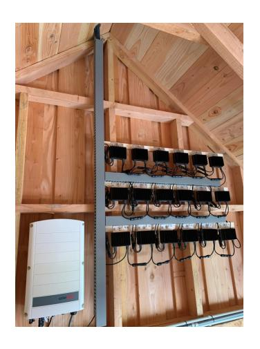
The Sunslates are electrical connected to the grid as a normal PV system.
