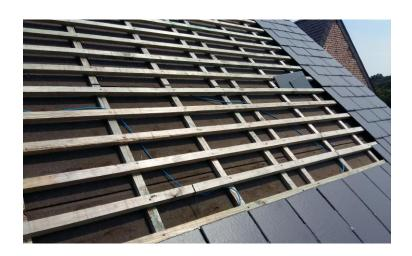
The **Sunslate** needs a tiling batten distance of **14.6** cm. Sunslate dimensions are 1140 x 400 x 5 mm. The overlap is 11 cm. The counter battens need to be minimum 20 mm heigh for good ventilation and let the connectors go under the battens while
