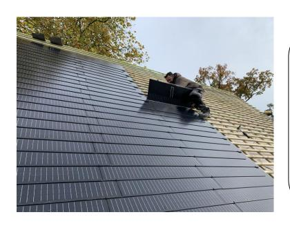
After placement of the tiling battens, each row is positioned on **1140.3** cm. After this we can prepare the solar cables on the under roof. We can connect one end of the string to the Sunslates and the other end inside the building to the Optimizers and inverter.
