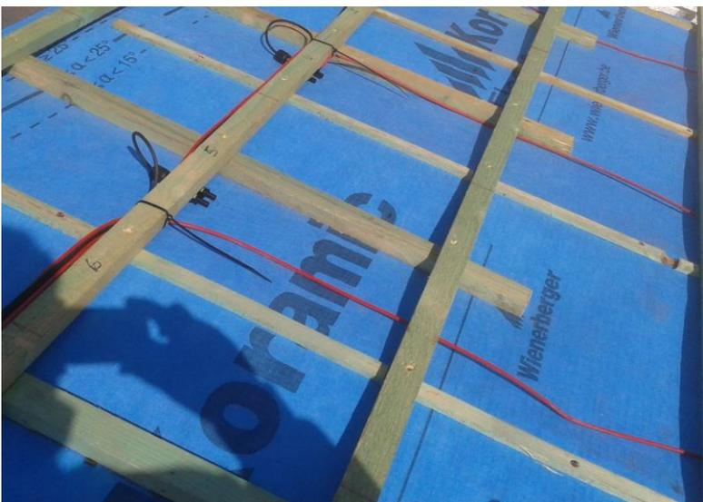
After placement of the tiling battens , each row is positioned on 35.2 cm (Cerasol) or 100.4 cm (Mini module). After this we can prepare the solar cables on the under roof. We can connect the sun tiles on one end and the Optimizers / inverter on the other.
