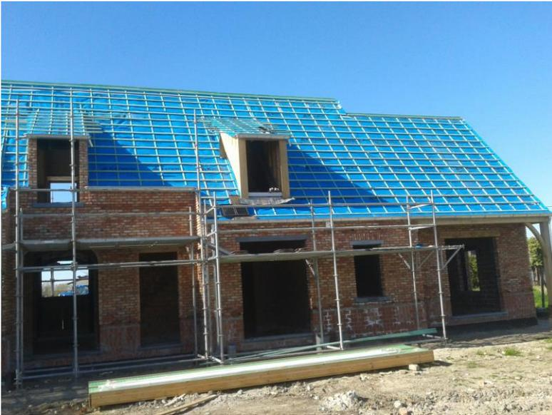
The Sun tiles from Smartroof are placed on a sloped roof such as the classic tile and can be installed during roof renovations and new constructions. No special underroof is needed.
