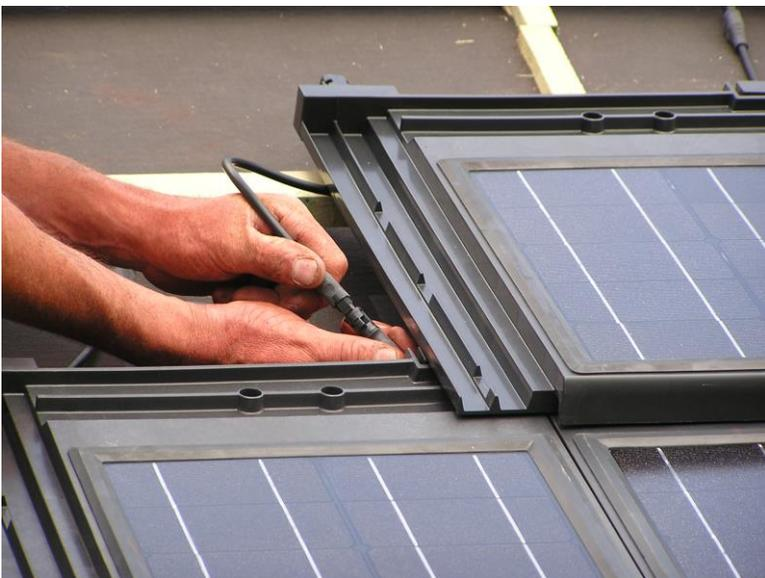
The electrical connection between the sun tiles is easy: just click in each other two MC4 connectors and connection is a fact! Each Sun tile has its own bypass diode.
