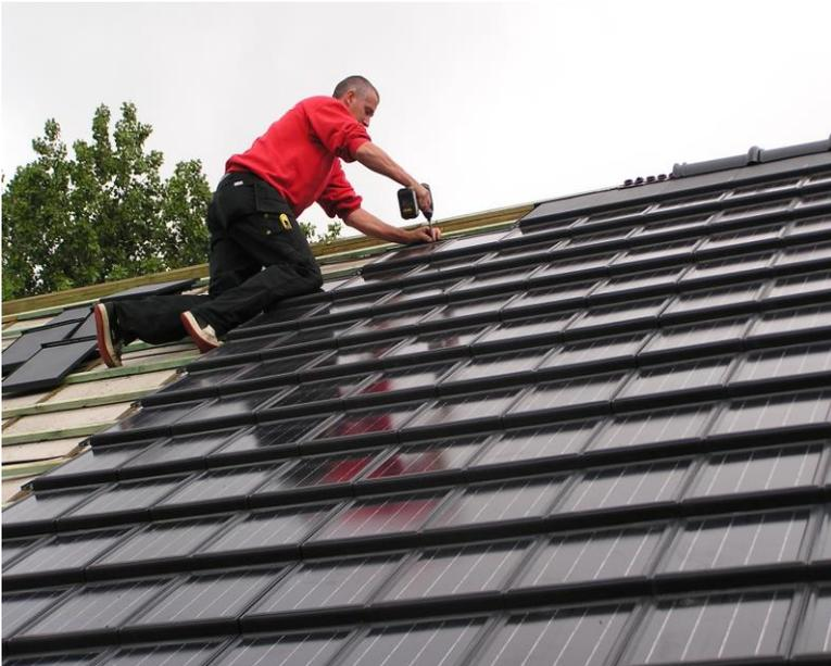
Each tile is fixed with a stainless steel screw on the tiling batten. An integrated hook makes that the tiles are holding nicely each other and making the roof homogeneous, airtight and weathers the storm. Total weight of the system is only 16 kg/m<sup>2</sup>!
