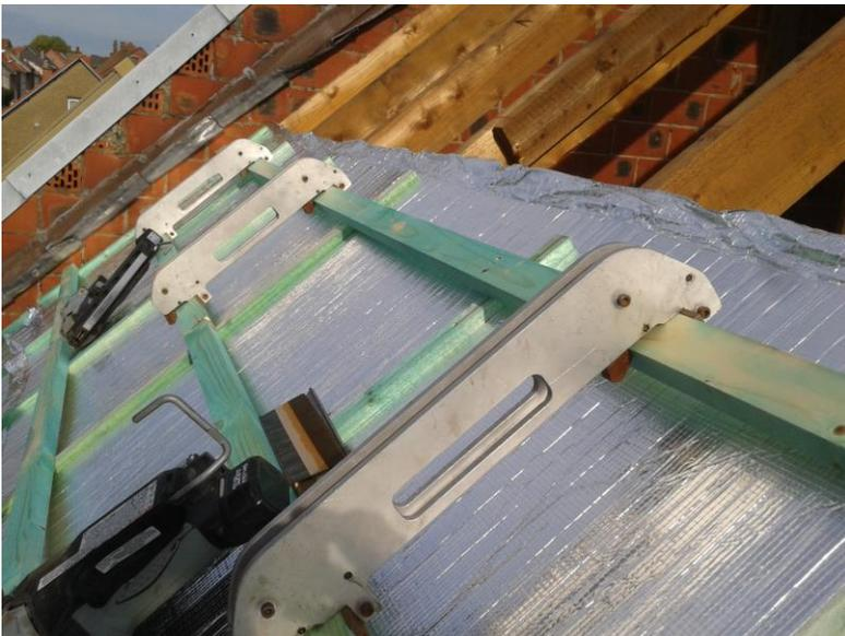
Calibres facilitate placing the tiling battens and guarantees a correct distance. The **Cerasolpan** and **Mini module** needs a distance of **40 cm** between the tiling battens, Neosolpan 35.3 cm and the RenoSolPan 24.6 cm.
